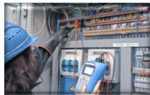
Switchboard testing
