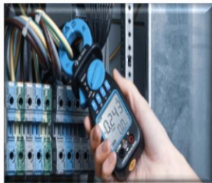
Electric Panels testing
